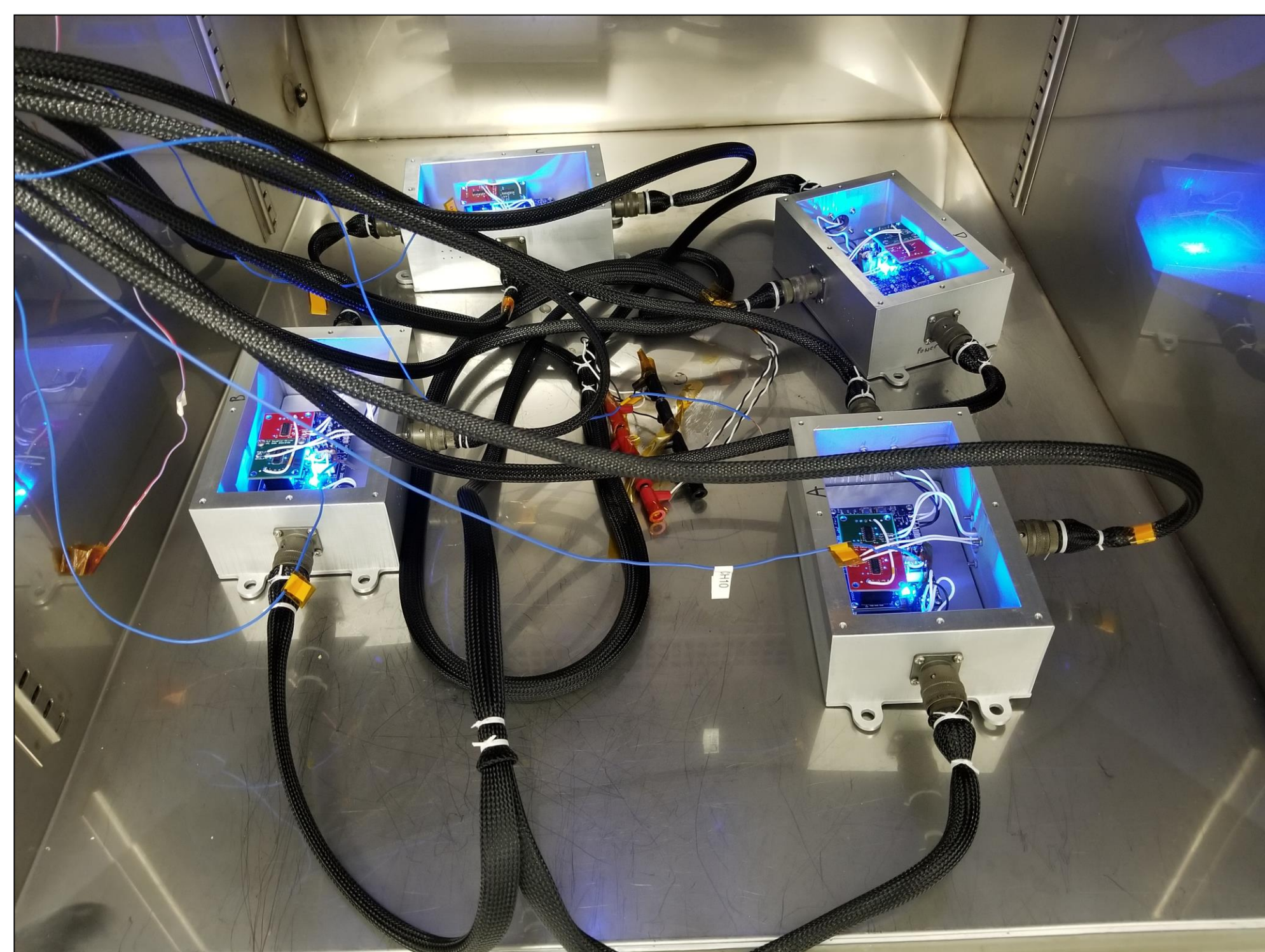
PLC Prototype Thermal Ambient Test Setup
