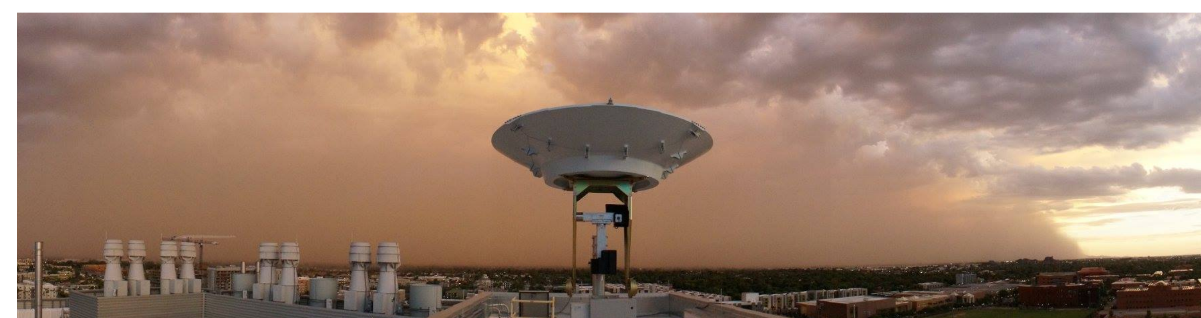
Figure 5: Dust storms pose great risk in the Phoenix metro area. Storm winds can reach 30 mph. The dish, positioned on the roof of an 8 story building, requires supplemental mechanical safeguards to ensure damage does not occur on the ground station gearing system. "birdbath mode" is used during storms to reduce the wind pressure on the dish.
