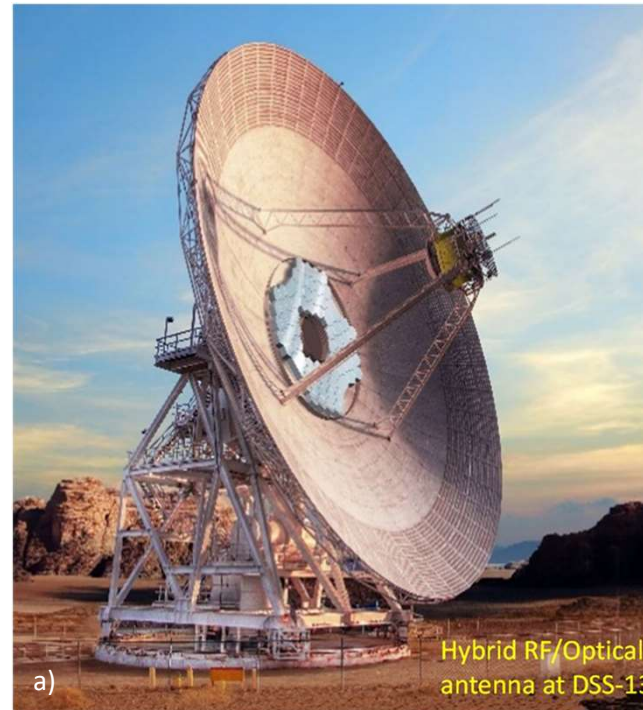
Figure 1. Main components of the Lunar Testbed deep-space channel emulator: a) hybrid RF/Optical receiver at DSS-13, with equivalent 8.3 meter effective optical collecting area; b) schematic of Apollo 15 lunar retro-reflector assembly, showing the layout of the 300 corner-cube retro-reflectors; c) diagram of a flight transceiver optical tube assembly (OTA).
